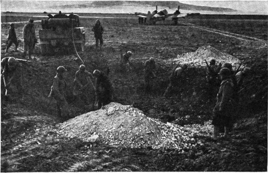
Figure 196. Pneumatic tamper compacting loose earth in bottom of bomb crater.
